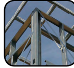
STEEL FRAMING CONTRACTORS
