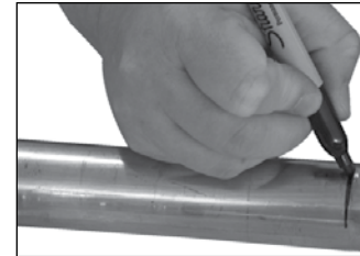
Figure 3 — Marking for Insertion Depth
