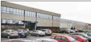
Montreal, Canada Velan Inc., Plant 1 and 5
