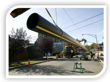
YELLOWSTRIPE<sup>®</sup> HDPE 8300 series is manufactured to meet your needs in compliance with ASTM D2513, NSF Gas and DOT 49 CFR 192. Selected sizes conform to CSA B137.4 and UPC product standards.
